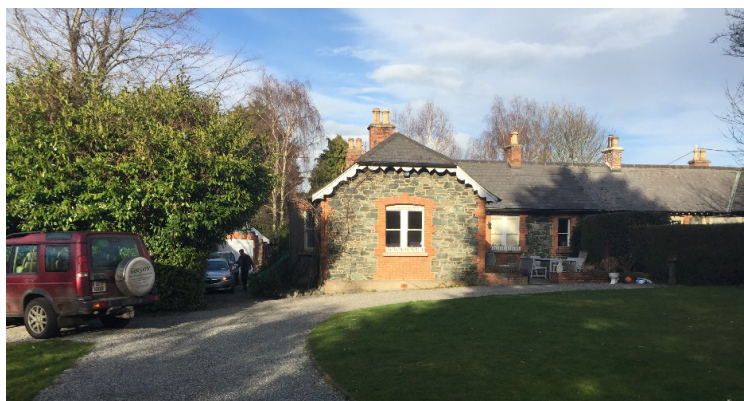
Greystones case study site, showing front aspect of the building and location of the ground heat exchangers in the driveway to the left of the house
