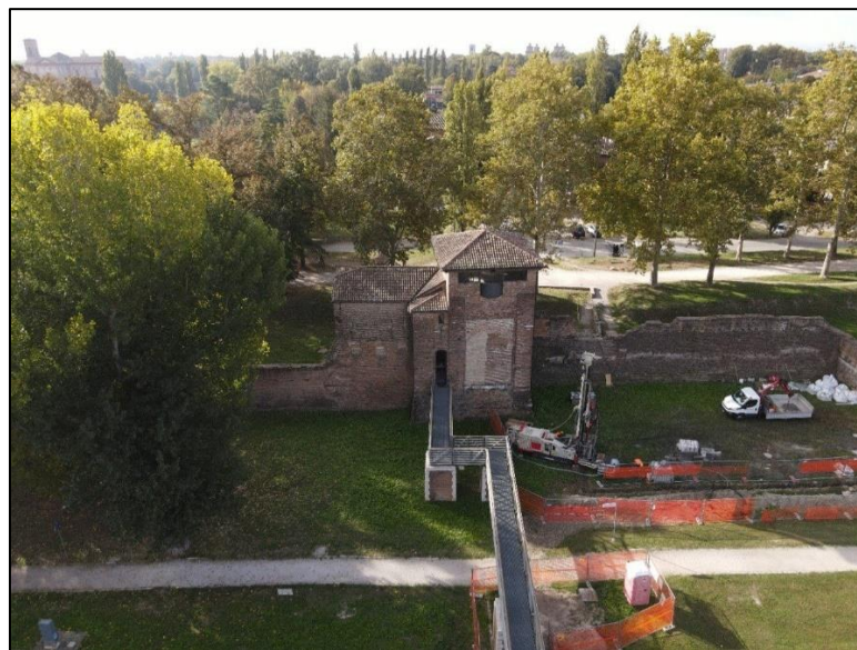
Figure 66 -Installation Example by GEO4CIVHIC (Porta Degli Angeli Ferrara, Italy)
