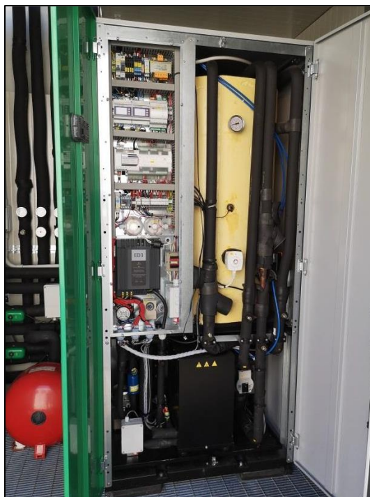
Figure 4.4 Plug and Play fixed-speed compressor (on-off, Prototype #1) and variable-speed compressor (inverter, Prototype #2) heat pump.
