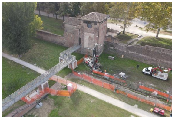
Figure 5: Aerial view of the geothermal field of Angel's Gate (Georicerche srl copyrights)
