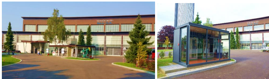
Figure 1: Nikola Tesla Technical Museum in Zagreb (left) and technical room devoted to the geothermal plant (right)
