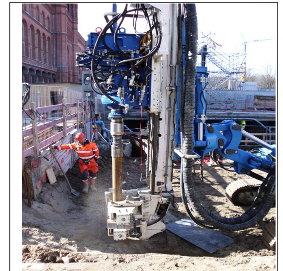
Vibration/rotation drilling head mounted on drilling rig
