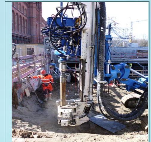
Vibration/rotation drilling head mounted on drilling rig
