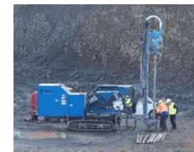
Rig with Vibro-Drill at Alsfeld test field
