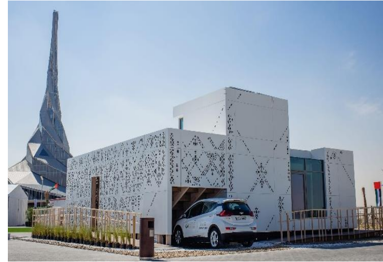
New EFdeN house built in Dubai (on wooden structure) – Solar Decathlon Middle East 2018 (to be relocated to the faculty's campus)
