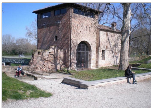
Figure 8 - Renovation of exterior space with pavement, grass, and benches
