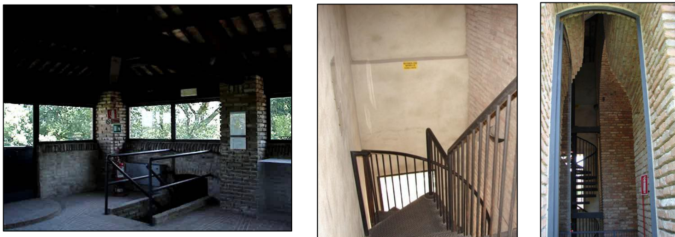
Figure 7 - Restoration of watchtower with shatterproof glass, addition of spiral staircase
